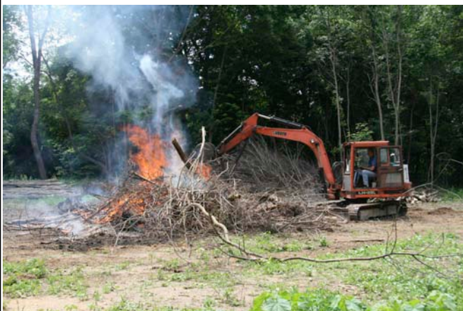
Ed Vanders starting the burn pile from the tree clearing.
